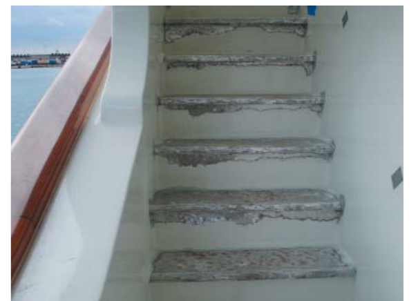
At the start of diary (top two images); Work in progress....
